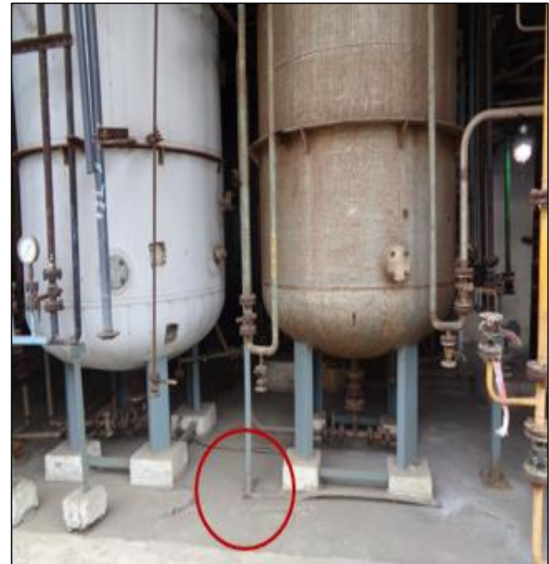
Static Double Earthing System
