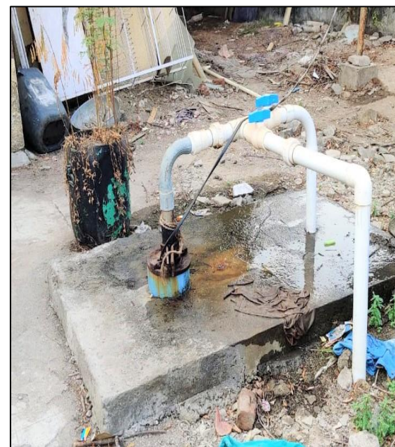
Injection system to Dry borewell
