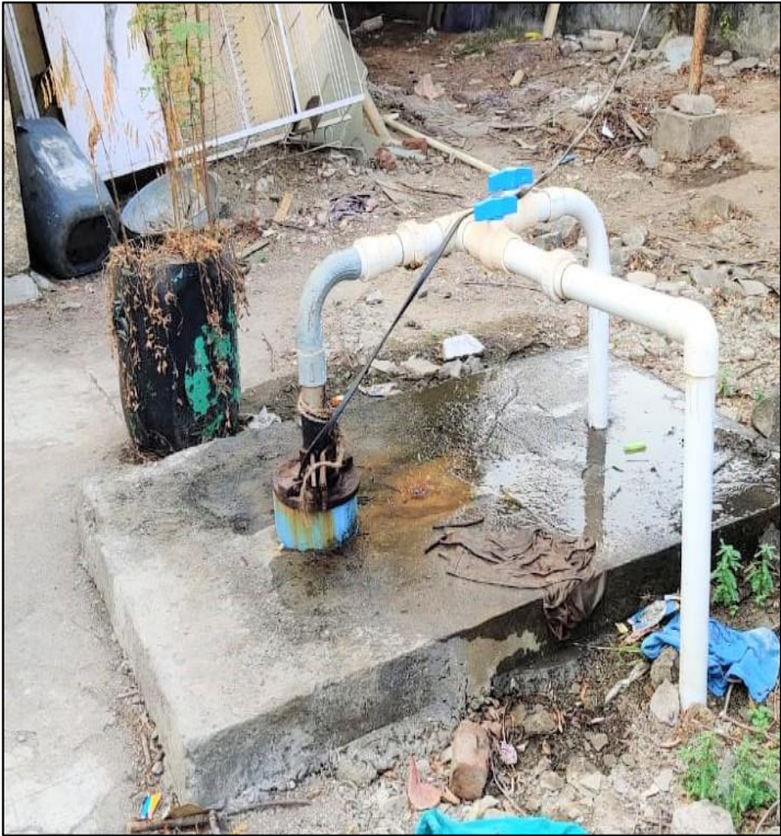
Injection system to Dry borewell
