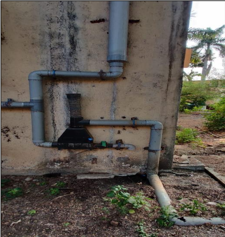
Roof water collection system
